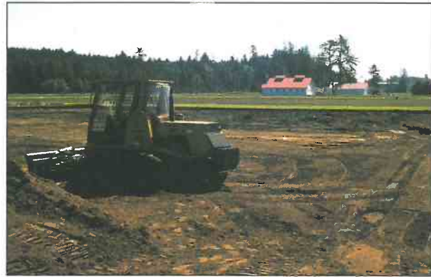
Figure 3.—Leveling returned topsoil on a bed.
