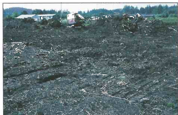
Figure 2.—Clearing land for cranberry bed construction.
