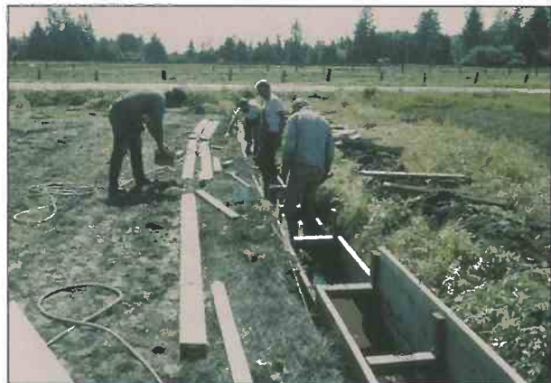
Figure 5.—Drainage ditch being leveled with pressure-treated wood and lined.
